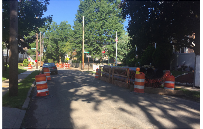
A view of the construction along Waters Avenue.
